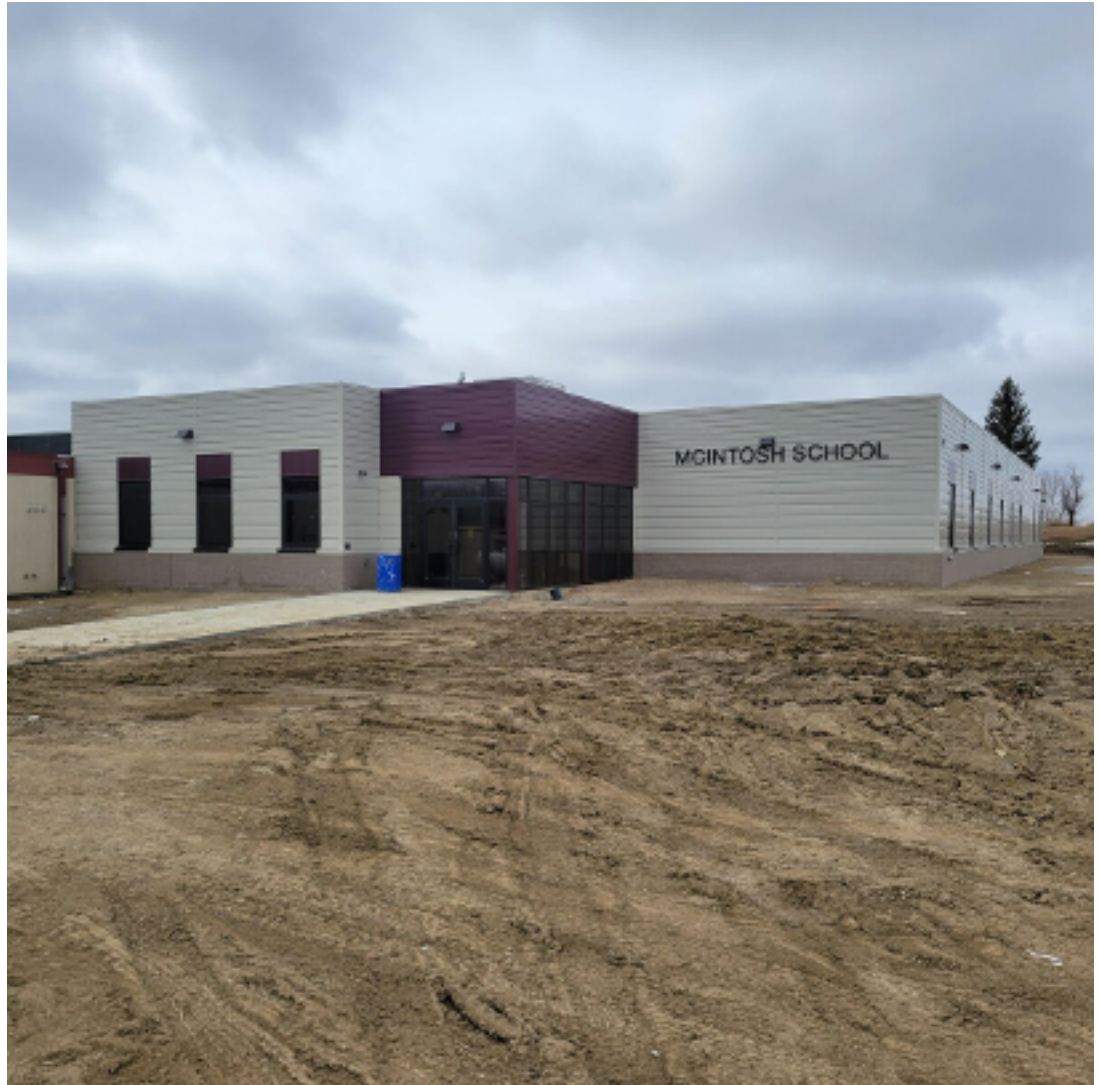
Construction underway on the McIntosh preK-8 school which opened in August 2025. Photo courtesy of McIntosh Public School.
